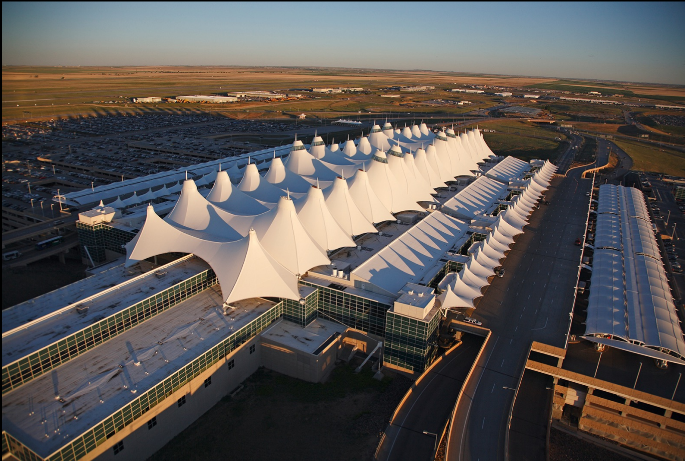
Denver International Airport, master plan and schematic design of the architecture with Perez Architects P.C. Summer 1988
